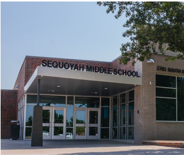
Sequoyah Middle School was renovated to better serve its students.
