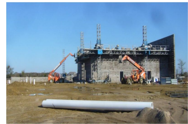
Oneta Ridge in Progress
